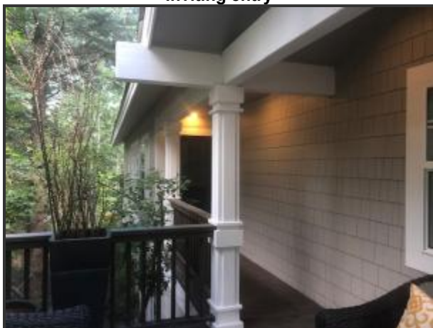
Inviting entry with wooden decking, room to sit and a sophisticated Navy Blue Door!
