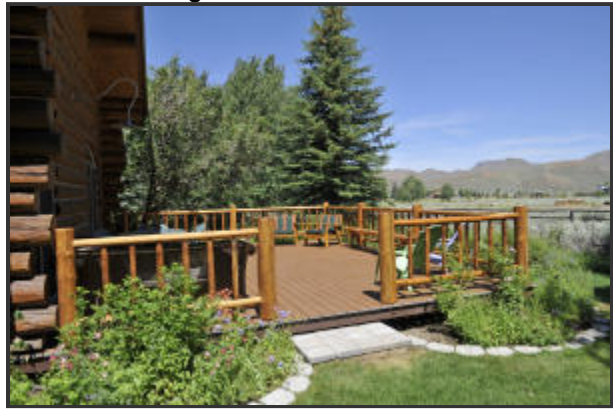
W facing deck off of the Great Room
