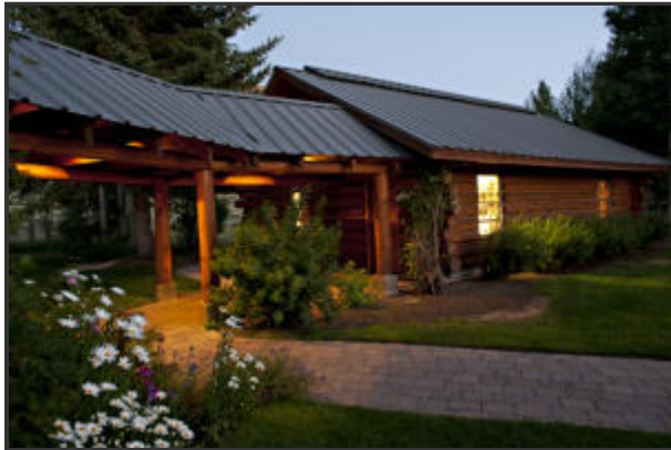
43 Pioneer View Dr. Covered walk between garage and home.
