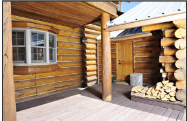
Kitchen window look out onto the patio and S facing back yard.
