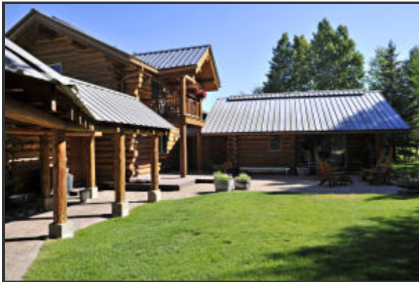
Back Yard from garage looking towards to house
