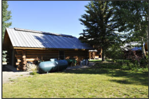
Garage w/ Propane
