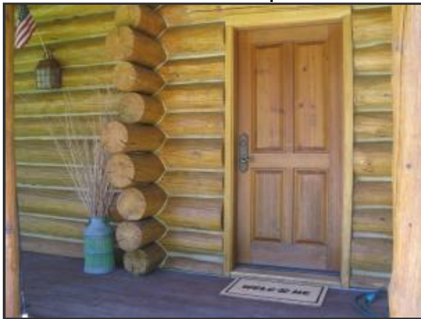
Front door covered porch
